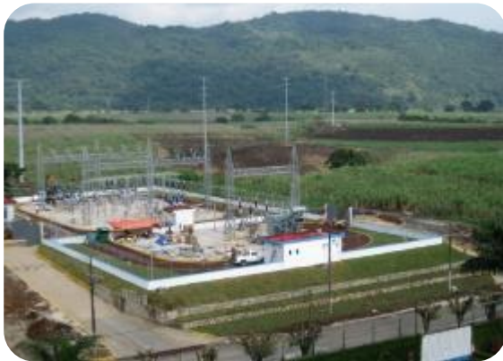
Areal photograph showing the final construction
